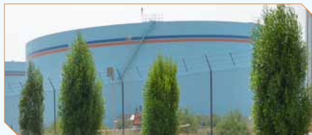
Figure 2: Potable water storage
